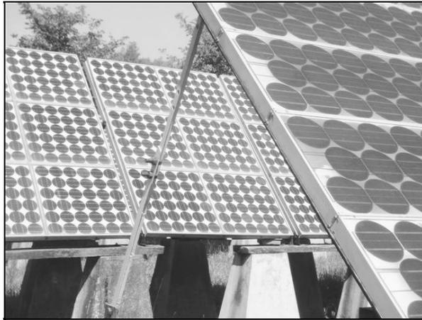
**Figure 3:** Photovoltaic array with variable modules inclination angles
