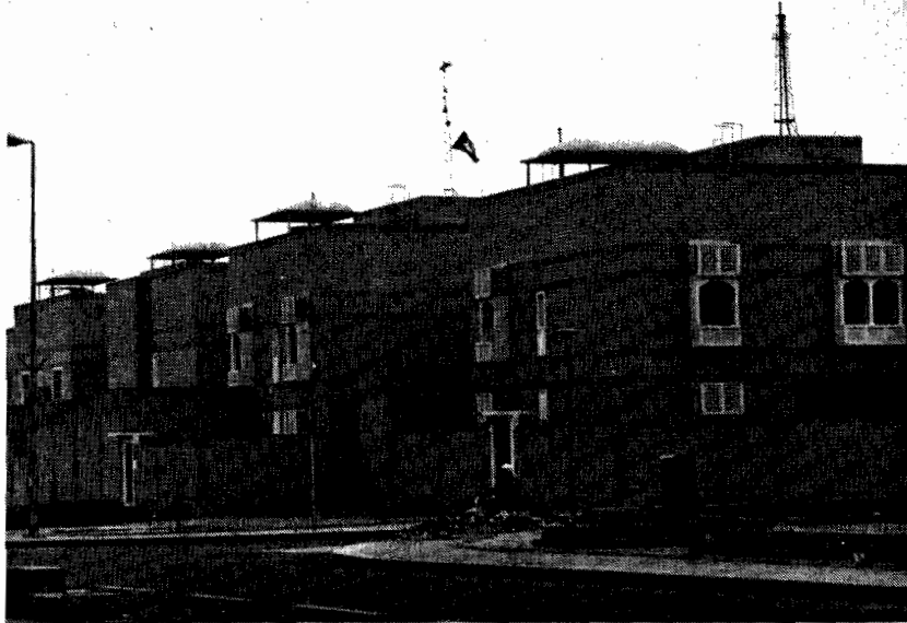
Fig. 2. A typical NHA housing project
